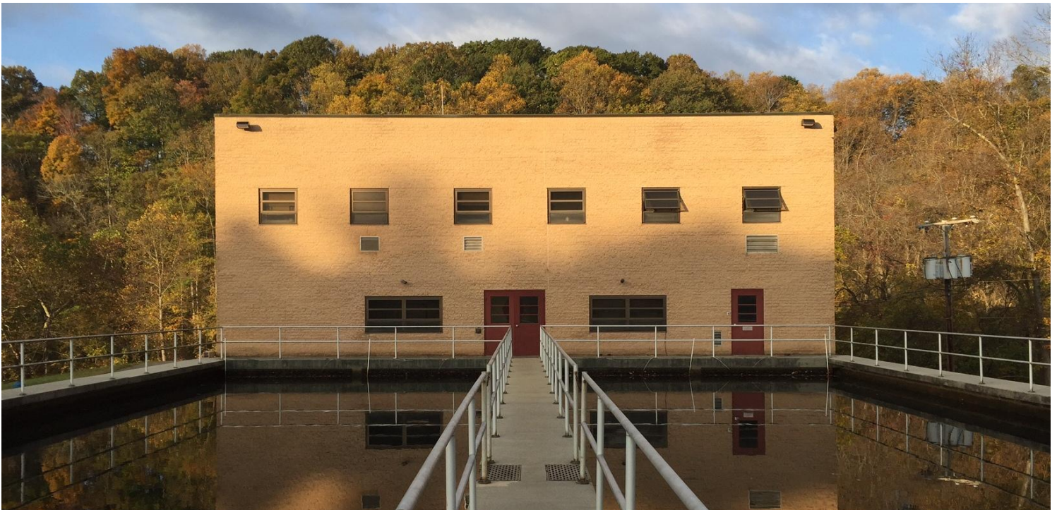
A view of our twin settling basins. This is where most of the particulate matter is removed.
